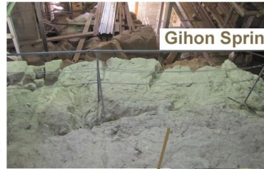
Natural Tunnel Blocked
