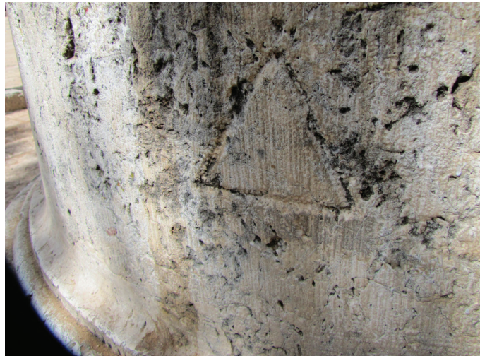
The Roman inscribed Delta which represents the number 4. This would have been the fourth column in a series of columns.
