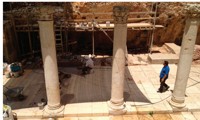
A nice view of the excavation revealing the street, the curb, the columns supporting the colonnade, the pedestrian sidewalk and the shops along the sidewalk under the colonnade.
