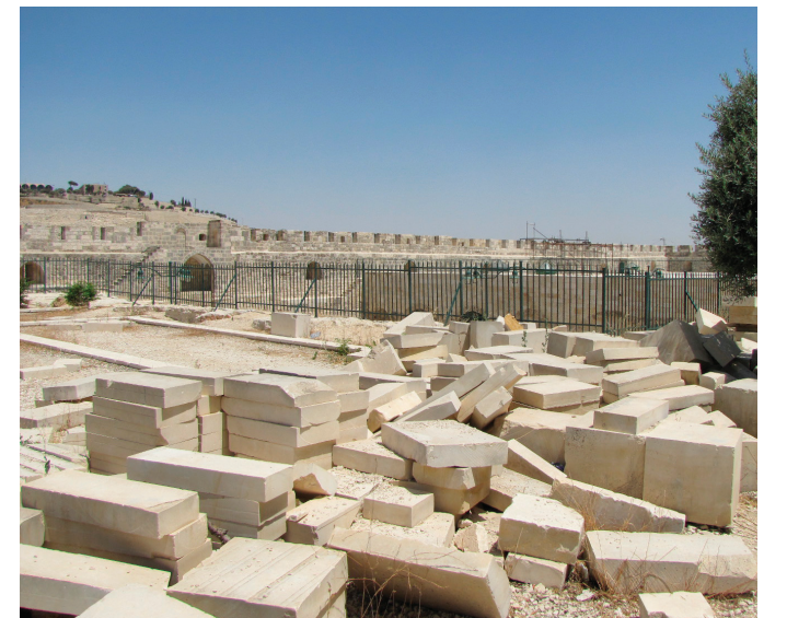
A supply pile of construction material still lies outside the fence near the new staircase down into the new mosque.
