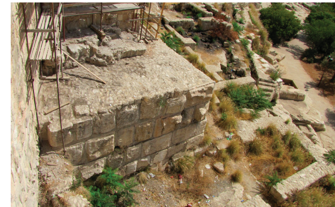
Photo of the outside the southeast corner of the Nea Church, which contains the southern apse of the church on the inside. The current city wall runs on top of the Nea Church, as can be seen in this photo.
