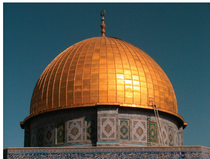
The dome on the Dome of the Rock was covered with an aluminum and bronze alloy in 1960. In 1998 it was covered with 176 pounds of gold (the value in 2010 dollars was $3,043,087) that was donated by King Hussein of Jordan. The diameter of this dome is 66 feet compared to the 69.5 foot width of the dome on the Church of the Holy Sepulcher, which the builders attempted to imitate. This dome is 67 feet high, and the dome of the Holy Sepulcher rises 69 feet.
