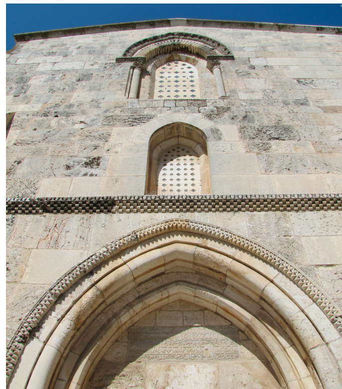
The windows and arch on the front of the church. The arch reaching a point at the top makes it a typical Crusader-style arch. Note that Saladin's 1192 inscription is under the arch.
