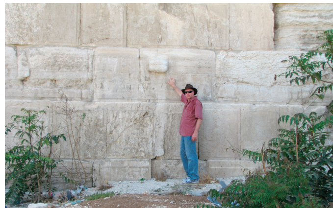
Galyn points at a projection left on an ashlar. These rock projections (one on both sides of the block) would have served as handles for the workers to attach ropes in order to pull and then lift the ashlar block into place. Several ashlars on the south and east side (particularly in the southeast corner) of the Temple Mount can still be seen.
