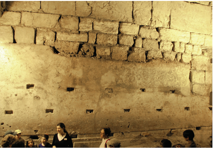
The Master Course Stone: This stone is 44 feet long, 11.5 feet high, and 15 feet wide. It is estimated to weigh 570-630 tons. This stone is the master course. It was used to stabilize the smaller stones under it. It sits 20 feet above the Herodian street level and 33 feet above the bedrock. The master course extends to the left of the edge of this photo and past the right edge. The small stones set above were used to fill in where the Romans chipped away at it in 70 AD, while attempting to dismantle the whole Western Wall. They reached the level of this Master Course Stone and stopped. The rectangular holes in the stone were bored centuries later to help secure plaster to the wall in order to create an underground cistern to hold water for the homes above.
