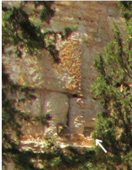
A close up of one of the 19-inch square sockets cut into the Temple Mount that was used to support a wooden beam that sat on the columns and served as part of the roofing structure in the colonnade.
