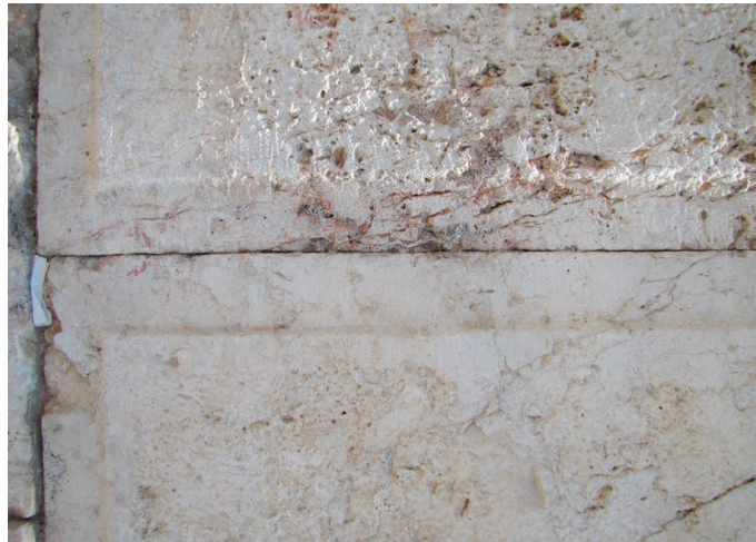
The tight horizontal joints of ashlars sit on top of each other in the Temple Mount wall.
