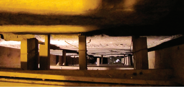
This photo was taken from the tunnel along the Western Wall looking down into an excavated area of the wall. (The Western Wall is at the top of the photo.) This view shows how deep the courses of ashlar stones go before they reach bedrock.
