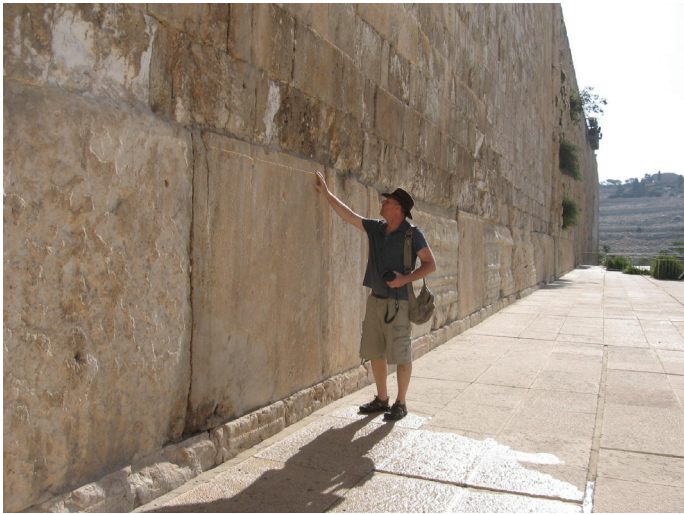
Galyn touches the carved top margin of one of the six foot tall Herodian ashlar in the master course of large stones. This stone is set on a smaller course of three foot tall Herodian ashlar. The Mount of Olives is in the background to the east.
