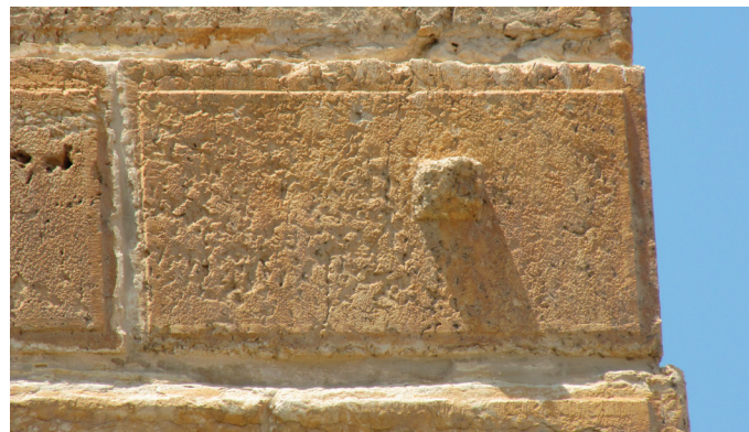
This is a Herodian ashlar stone on the SE corner of the Temple Mount retaining wall in Jerusalem. The protruding square knob on the side was used for attaching ropes to pull and position the block into place on the wall. Once the block was set in place this knob was usually removed by the stonemasons.
