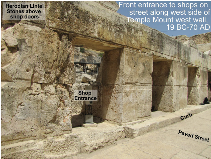
A close up of the front of the shops sitting along the Herodian road. Notice the nicely cut ashlar stones that formed the door jambs and supported the lintels above the doorways. This street was lined with shops on both sides.
