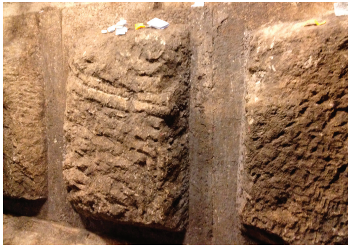
Ashlars with unfinished bosses near the base of the retaining wall are still set perfectly in place with their tight vertical joints, 2,000 years after having been set in place. Also, notice the course of ashlar stones is set back about 1/2 inch. This 1/2 inch set back continued all the way up the wall to help stabilize the stacked stone wall.
