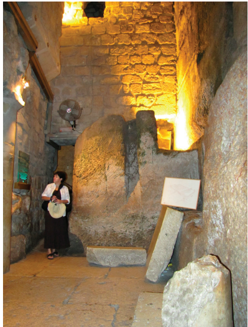
Toni stands by an unfinished quarried stone. Wooden blocks would have been wedged into the groove in the middle and then soaked with water to make the stone split.
