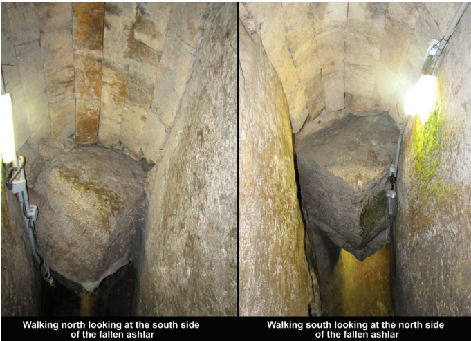
A photo from 2012 of the same gutter with the same fallen ashlar stone protruding through the ceiling under the pavement of the Western Wall road.
