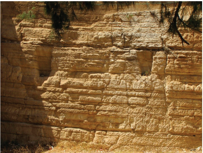
This is a photo of the trapezoidal sockets cut about 9 feet high in the bedrock. They were cut between 650 and 900 AD by Muslims to support wooden beams for one of the roof systems in their buildings.
