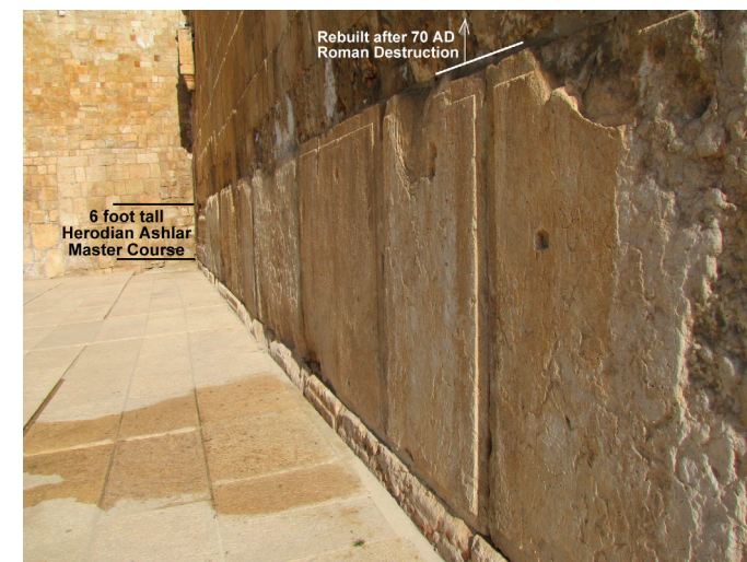
These ashlars along the southern wall of the Temple Mount between the Double Gate and the Triple Gate are twice the height of the other Herodian courses. These were a stabilizing band known as the great course.
