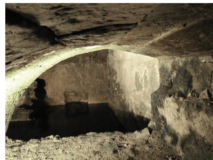
This is one of the vaulted arches built in 135 AD to cover this open aired Struthion Pool. The opening or hole seen in the top of the arch provided access from the pavement above to the water below by lowering a bucket on a rope.
