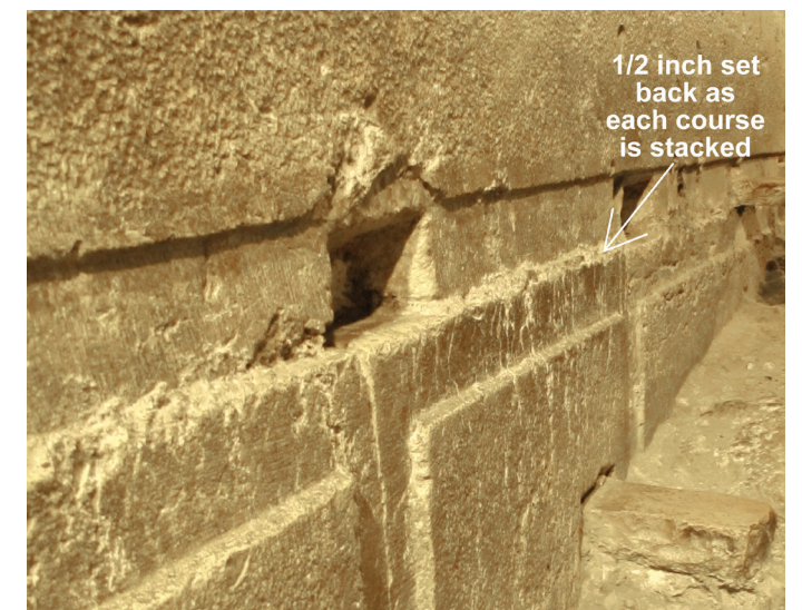
The stone on the top is the Master Course Stone found in the Western Wall Tunnels. Notice again the 1/2 inch set back as each course is stacked on the other. We will see more later about this stone, possibly the largest stone in the Temple Mount wall. The rectangular notches were cut at a later time when this wall was used as part of an underground cistern. Plaster needed to be applied to the entire cistern in order to make it watertight. Holes were cut in the stones to keep the plaster attached, and long stones were placed in each hole. The plaster was then applied to the wall. In this photo you can see the Herodian Ashlars, the rectangular holes, the long brick-shaped stone placed in the hole, and a very thick layer of plaster attached to the ashlars and strengthened by the stone connector.
