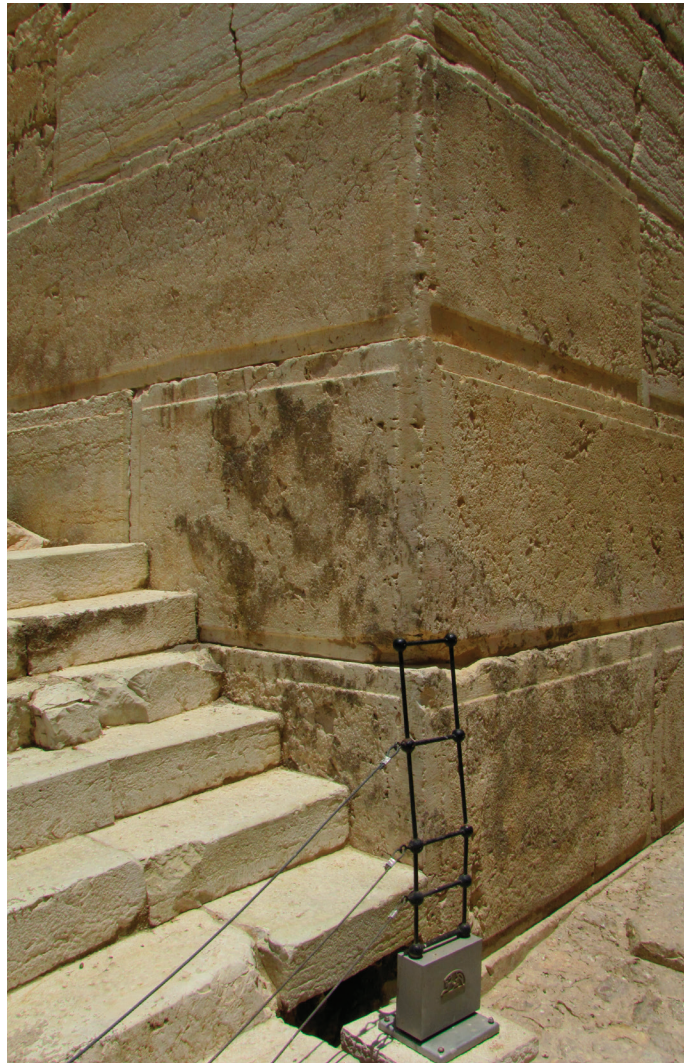
This photo shows the southwest corner of the Temple Mount wall. The Herodian ashlar cornerstones are clearly visible. To the right (east) are the pavement and steps that lead along the southern wall. To the left (going north) are the stair steps that led up to the top of the shops that sat along the Western Wall.
