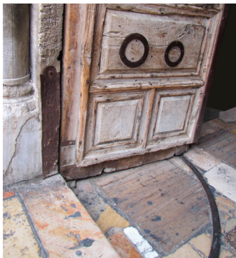
Photo of the left door showing the tracks on the floor that the door moves on.
