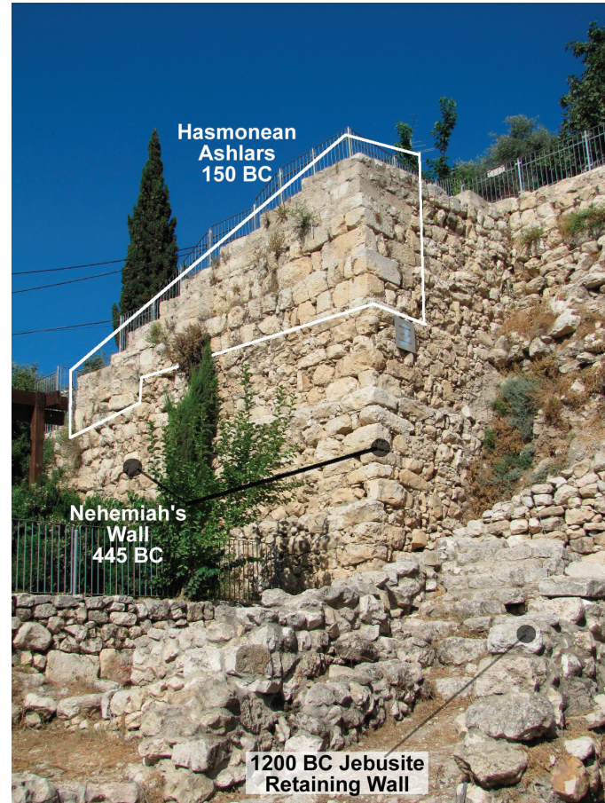
The tall straight wall with the corner is a portion of Nehemiah's wall from 445 BC that the Hasmoneans re-built around 150 BC on the east side of the City of David. The Stepped Stone Structure is to the right in this photo. Some of the retaining walls from 1200 BC can also be seen in the bottom right of this photo.
