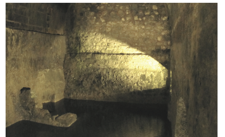
The openings in the vaulted ceiling that can be seen in this photo (and in the photo above) were used in Hadrian's time (around 135 BC) to access the water in these covered pools from the market square that was built above.
