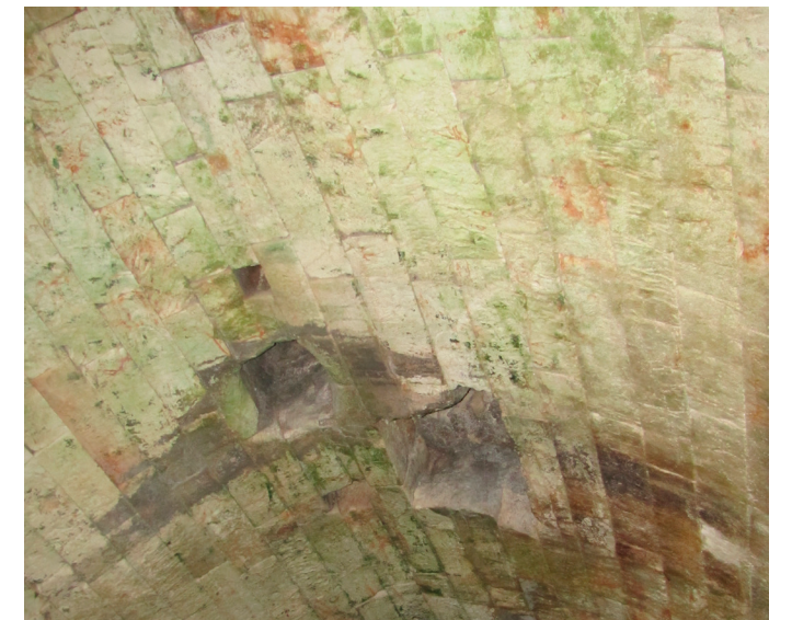
The openings in the vaulted ceiling that can be seen in this photo (and in the photo above) were used in Hadrian's time (around 135 BC) to access the water in these covered pools from the market square that was built above.
