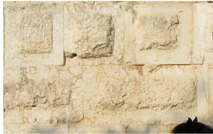
Notice the margins cut smooth around the edges and the rough boss in the middle decorating the face of each block.
