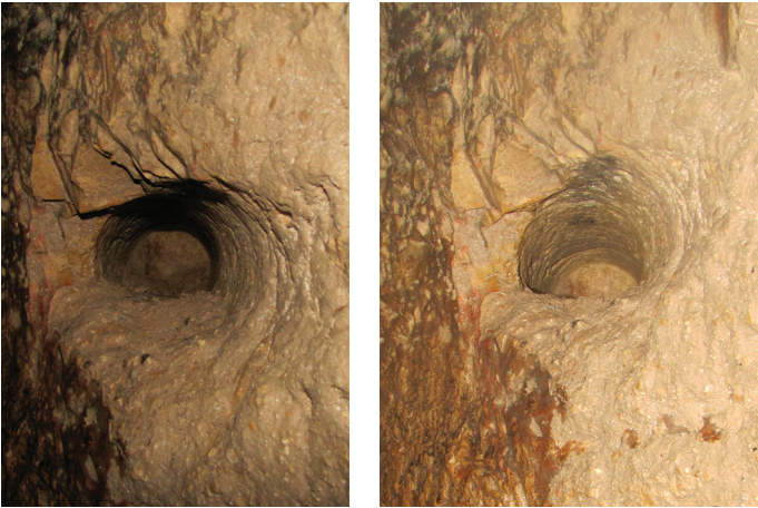
Holes in the walls were cut out by the workers to hold torches for light in the dark tunnel.
