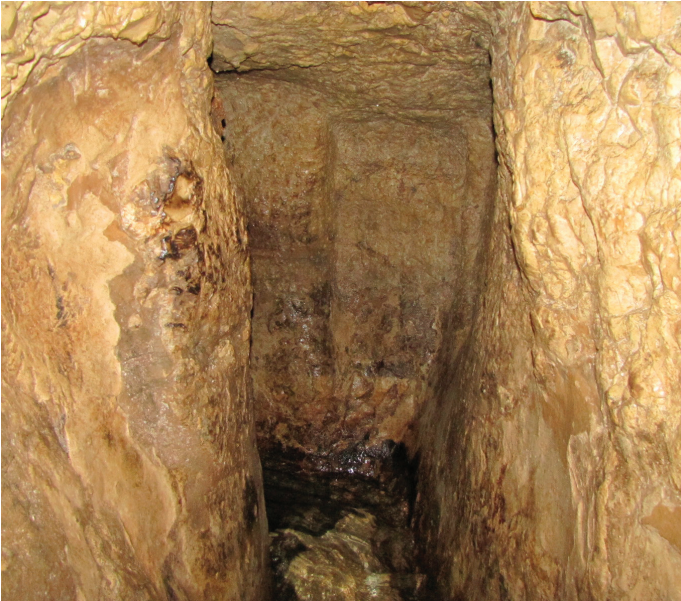
A bend in the tunnel going left (south toward the Pool of Siloam) was made as the two crews of tunnelers were trying to meet each other. In this photo the impression of the beginning of a straight tunnel can be seen in the tall, rectangular shape indentation. This direction was abandoned and the northern crew digging south from the Gihon Springs turned left. The meeting place where the two crews met occurs just around this corner after a few more false starts.
