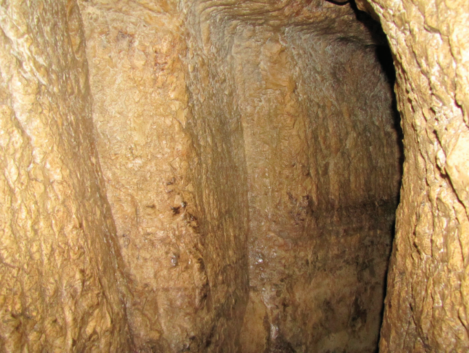
Here the tunnel weaves to the right after passing the point where the two crews would meet. False starts (i.e. the beginnings of wrong directions in the tunnel), made by the crew digging north from the Pool of Siloam can be seen in this photo by the marks on the walls. At this point the crews were attempting to meet each other so the water could flow from the Gihon Springs through the tunnel to the Pool of Siloam.
