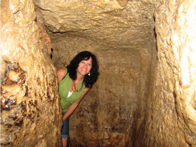
Toni coming from the south a few steps after the point in the tunnel where the two crews met. One of the false starts made by the crew coming from the north can be seen in the wall.
