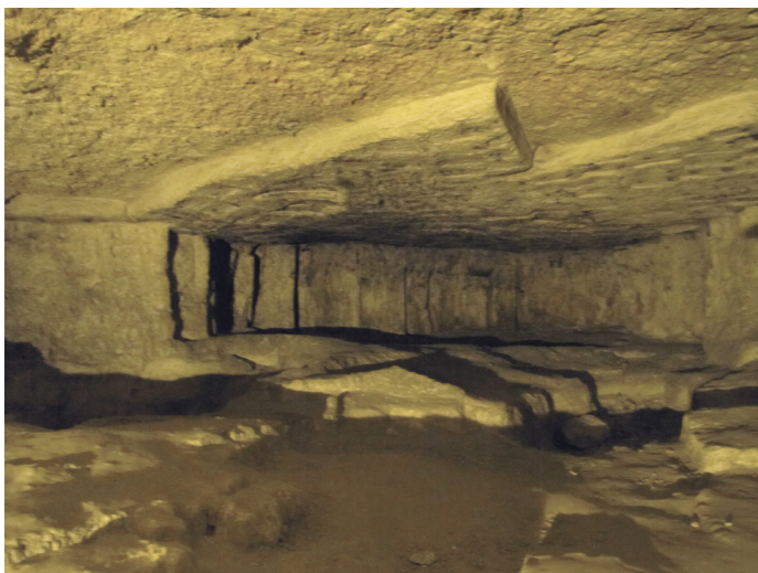
A section where the walls and ceiling show signs of the removed ashlars.
