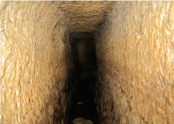
A nice photo of the tunnel clearly showing the pick marks, the sharp corners where the walls and ceiling meet, and the fresh moving, cool water on the floor of the tunnel which comes above the ankles to mid-calf.
