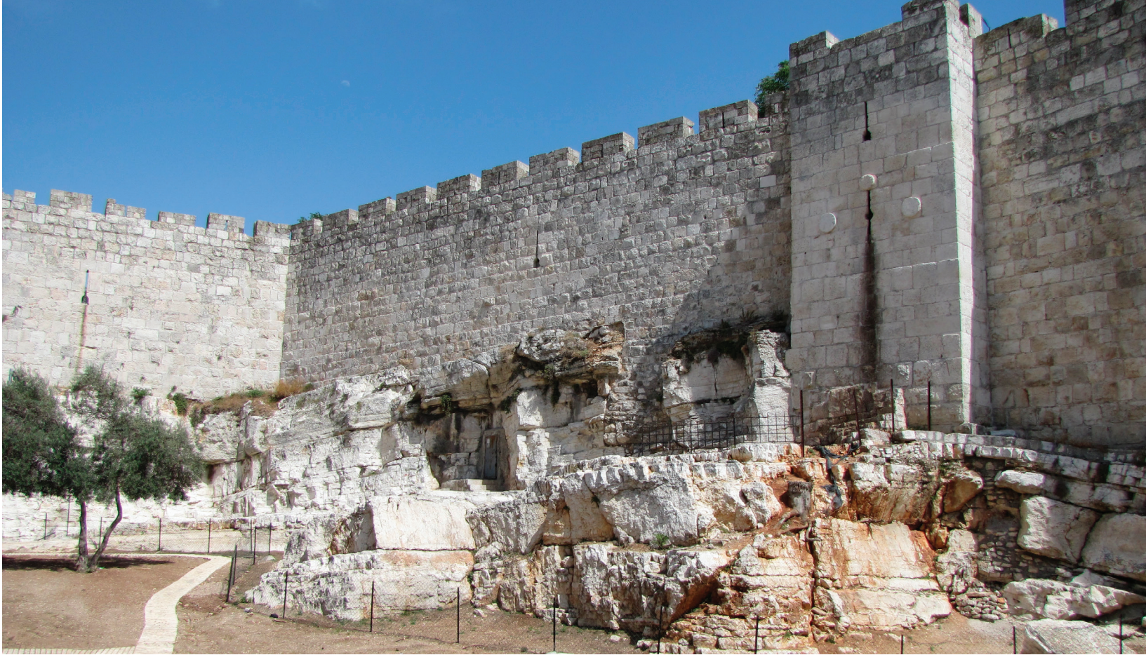
Part of the North Wall rests on the exposed bedrock of Mount Moriah.
