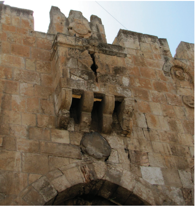
A machicolation, typical of castles and fortifications of the Middle Ages, where hot oil or rocks were dropped on the invading enemy below.
