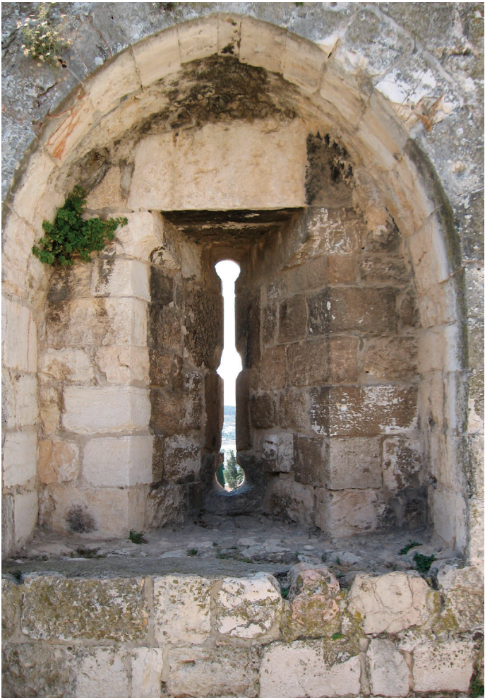
This is the inside view of the window in the wall above. Notice it is narrow on the outside to hinder incoming arrows, but wide on the inside to allow the archer to shoot from a wider range of angles at the enemy below on the outside of the wall.
