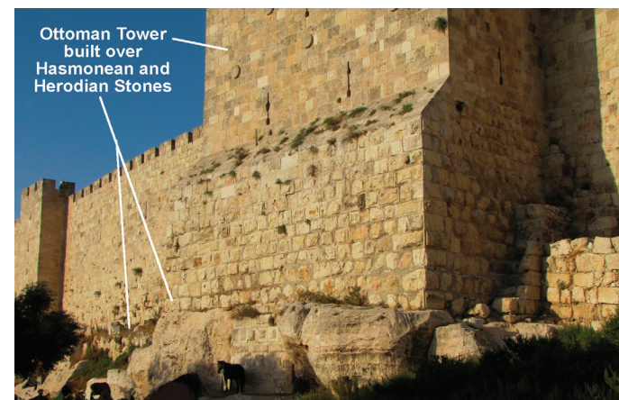
A Turkish, or Ottoman, Tower built by Suleiman. Notice the outcropping of the bedrock under the tower. The walls had to be built on solid bedrock and in many places this bedrock can be seen above the surface of the ground. Each period that built or rebuilt the walls tended to follow the same wall line along the bedrock.
