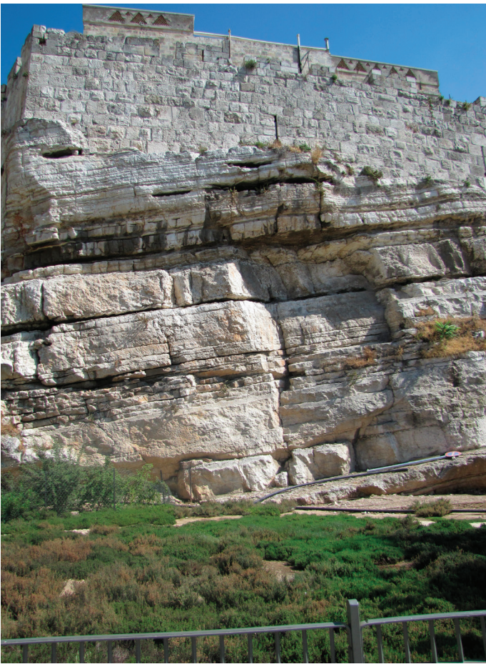
Much of the North Wall is built upon the bedrock protruding from Mount Moriah which continues to rise as it moves north through Jerusalem from the Temple Mount. The ancient walls of the city of Jerusalem also followed this exposed bedrock which means much of today's northern wall of the city is situated in the same location as the ancient walls of Jerusalem.
