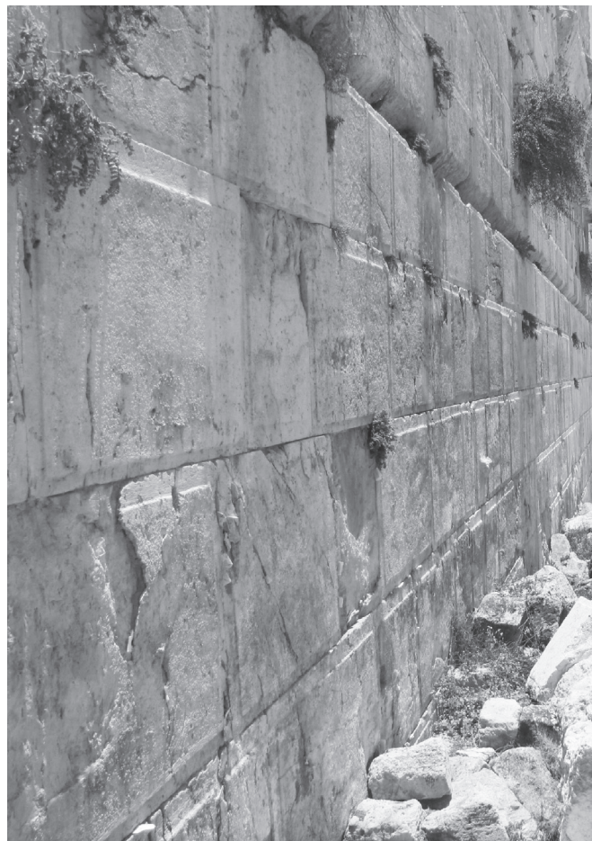
Four courses of original Herodian ashlar can be seen on the Western Wall of the Temple Mount.
