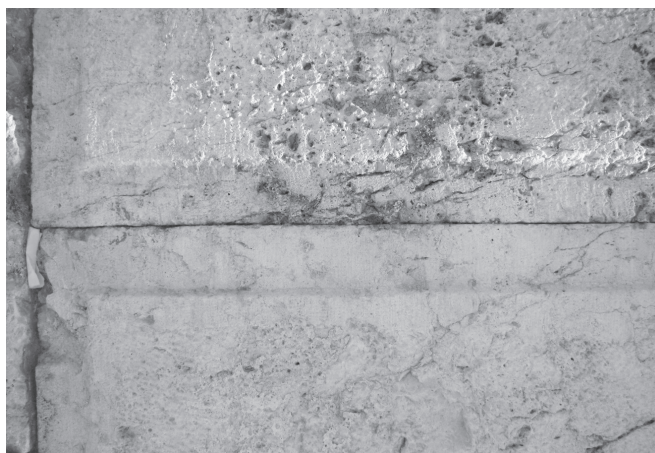
The tight horizontal joints of ashlars setting on top of each other in the Temple Mount wall.
