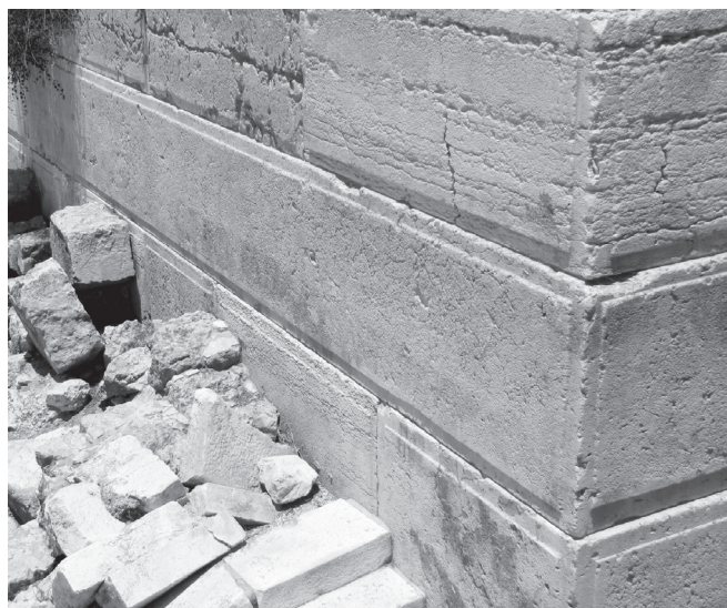
A very large corner stone with margin and boss, located on the southwest corner of the Temple Mount. This southwest corner has some of the largest ashlar stones of the entire Temple Mount complex, measuring 39 feet 4 inches long by 7 feet 10 inches wide and 43 inches high. The large stone shown here is called the master course stone and weighs about 80 tons. All these stones form a strong corner as they alternate back and forth as headers and stretchers all the way up. The larger stones helped stabilize the smaller stones stacked below.
