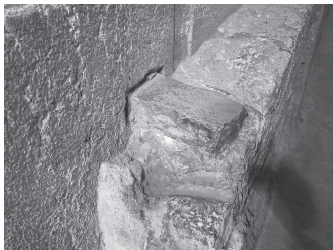
A close look at the ashlar with the wooden (stone) block holding the plaster in place in the Western Wall tunnel.
