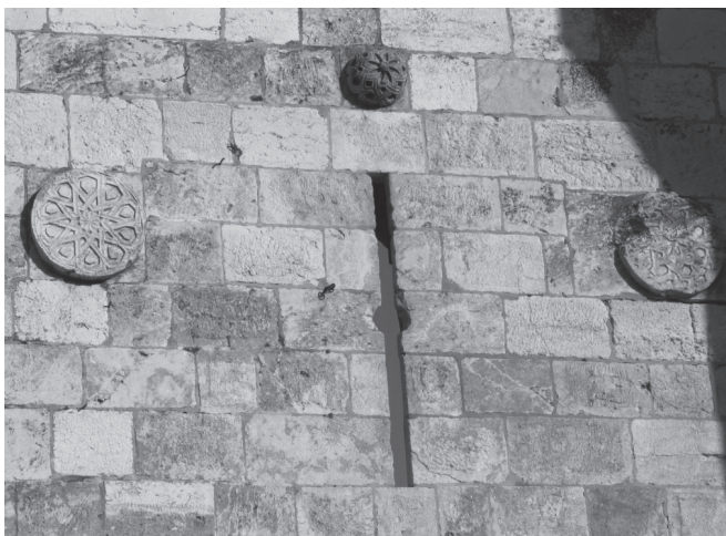
Arrows and bullets were fired from these loopholes, or arrow loops, which are narrow vertical windows in the wall.
