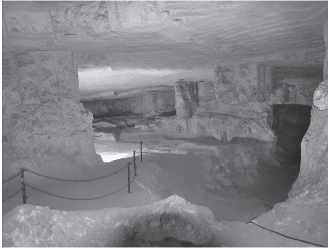
The stone ashlar were taken from this quarry. The straight cuts and grooves of the square blocks that were removed can still be seen.
