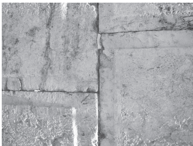
The margins, the raised bosses with the smooth face, and the tight joints in Herod's Temple Mount wall.
