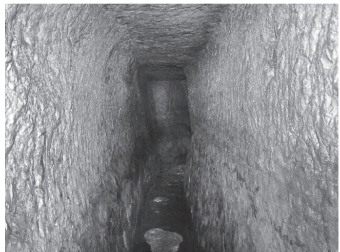
A nice photo of the tunnel clearly showing the pick marks, the sharp corners where the walls and ceiling meet, and the fresh moving, cool water on the floor of the tunnel which comes above the ankles to mid-calf.
