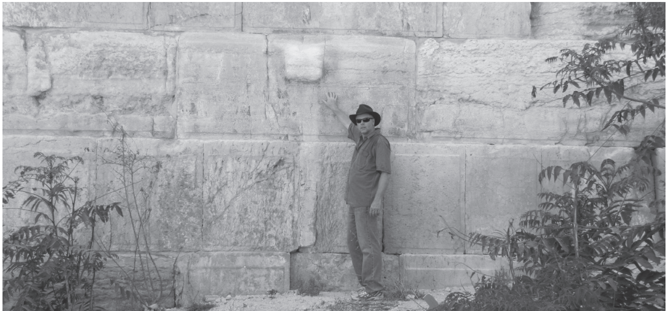
Galyn points at a projection left on an ashlar. These rock projections (one on both sides of the block) would have served as handles for the workers to attach ropes in order to pull and then lift the ashlar block into place. Several ashlars on the south and east side (particularly in the southeast corner) of the Temple Mount can still be seen.
