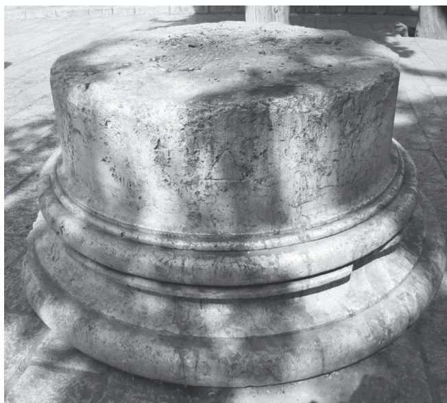
This is an Attic base of a Roman column next to the column above. The number 4 is inscribed on the second layer on the coved base as "Δ", which is the Greek letter Delta. The number indicates that this column base was the fourth in a row of columns. It has not yet been determined which building these columns belonged to.
