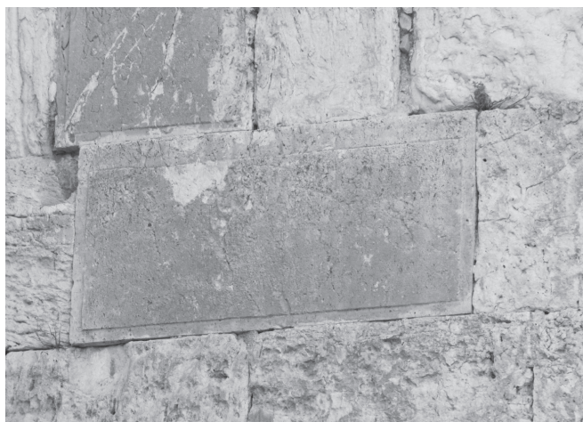
An ashlar in the eastern wall. Estimates by experts tell us that 200 workers could produce about eight cubic meters of cut stone each day. That means one cubic meter of stone ashlar would require about 120 hours of labor to cut and dress.
