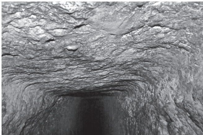
Detail of the ceiling that begins at about 5 feet high and ends a third of a mile later at 16 feet. Notice the pick marks of Hezekiah's men that can still be seen in the bedrock under the City of David.
