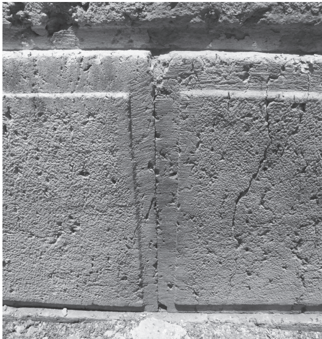
Details of the original perfectly tight horizontal and vertical joints. The workmanship of Herod's construction team still maintains its impressive quality, even after setting in the middle of all the wars and activities in Jerusalem for the past 2,000 years.
