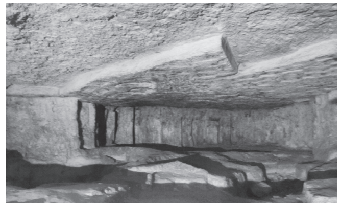
A section where the walls and ceiling show signs of the removed ashlar stones.
