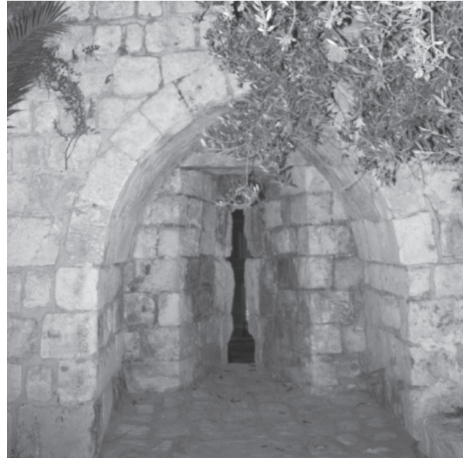
This is the inside view of the window in the wall above. Notice it is narrow on the outside to hinder incoming arrows, but wide on the inside to allow the archer to shoot from a wider range of angles at the enemy below on the outside of the wall.
