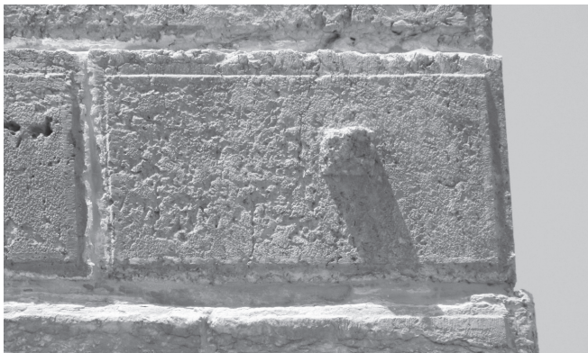
An ashlar and its uncut projection on the south side of the wall on the southeast corner.
