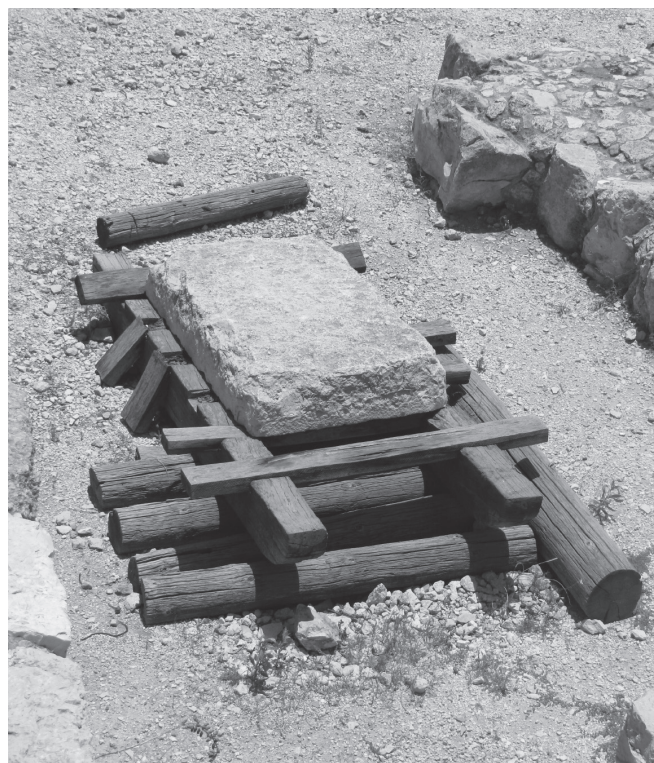
This is an example of a stone on rollers. The stone would be pulled by a team of oxen attached to a harness connected to the ashlar by projections of rock left uncut on both sides. On the next page are photos of projections left on the ashlar stones by Herod's workers.
