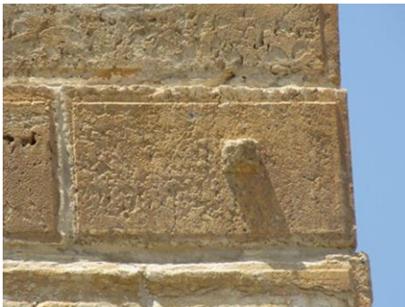
Herodian Ashlar with protrusion used for moving ashlar still attached.
