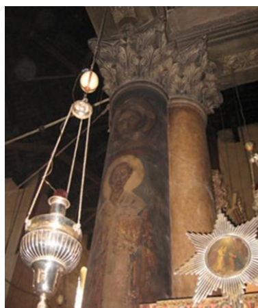
19.5' polished limestone columns of 325 AD with corinthian capitals covered with frescoes (pigment melted into wax) of the Apostles by Crusaders in 1100 AD
