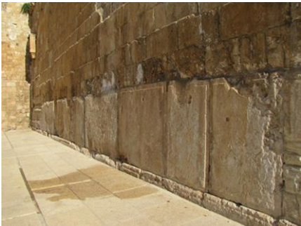
Large ashlar's in a master course in south temple mount wall.
